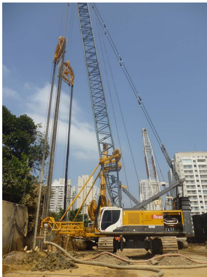
Figure 5. Excavation with hydromill
