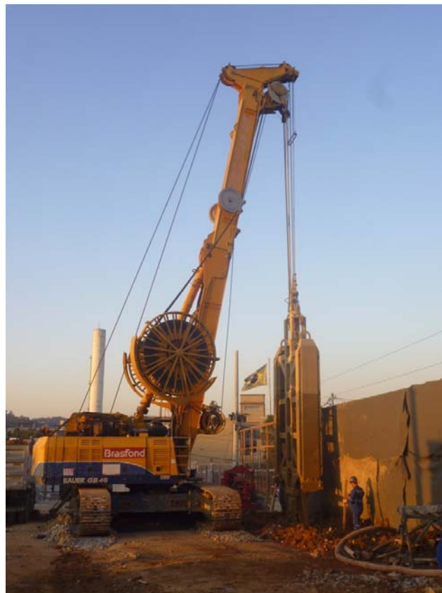
Figure 4. Partial excavation with hydraulic grab
