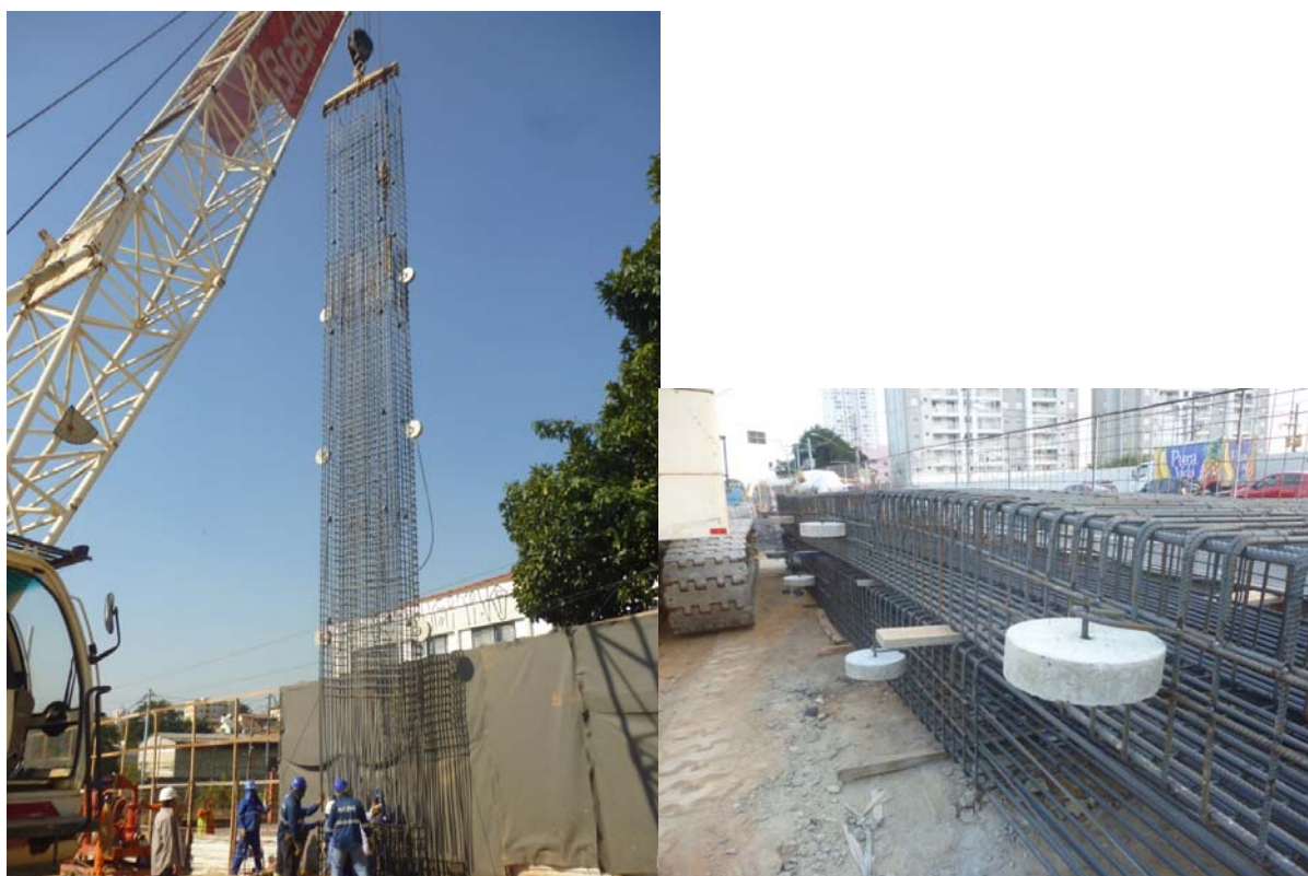
Figure 7. Placing the cage on the panel (left), using concrete spacers (right)
