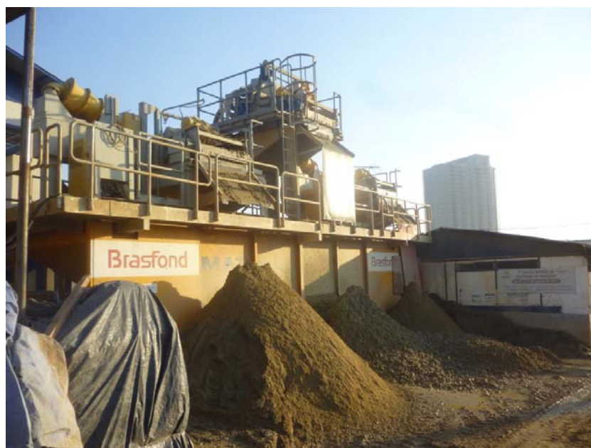
Figure 6. Desanding unit with excavated material
